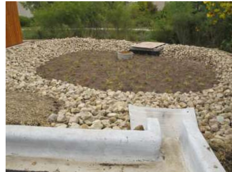
Bioretention with Sand
